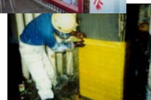
Retrofitting by FRP sheet
