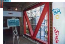
Retrofitting by steel brace
