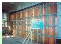
Replace brick wall to infill RC wall
