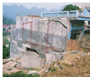
Damage to residences from landslides in Son La, the capital of Son La Province in Vietnam
