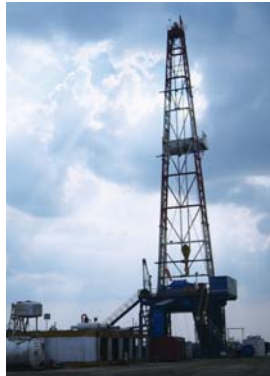
A drill rig in preparation for natural gas production
