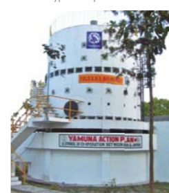
Prototype DHS plant in India
