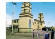
Church in the center of Pisco City that collapsed in the 2007 earthquake
